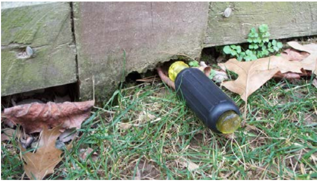
Deterioration failure of deck support post materials
