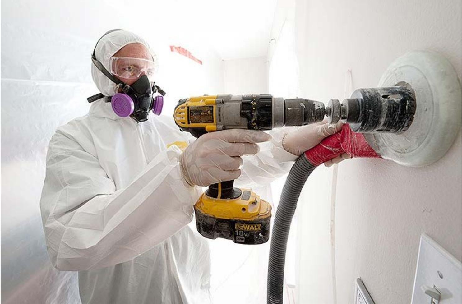
A weatherization worker drills holes to blow cellulose insulation in the interior walls of this home. | Photo courtesy of Dennis Schroeder, NREL
