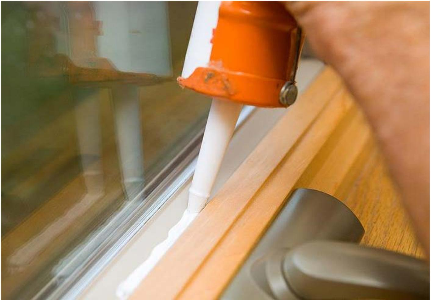
Applying caulk to a window frame to prevent air leakage. This caulk is white when applied, and dries clear. | Photo courtesy of ©iStockphoto.com/BanksPhotos.
